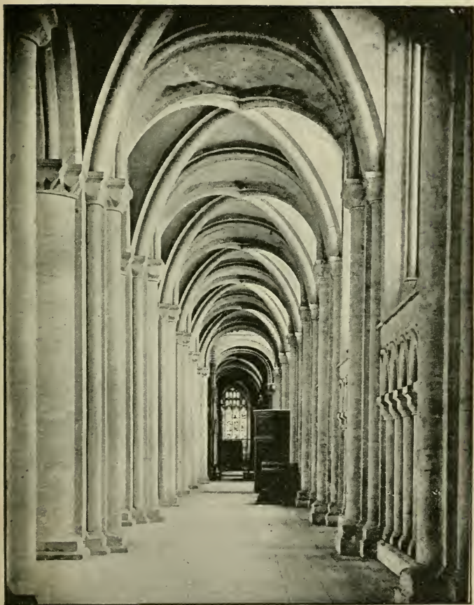
FIG. 78.—SOUTH AISLE. Peterborough.
